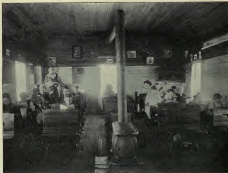
Interior, district 15, Salem
